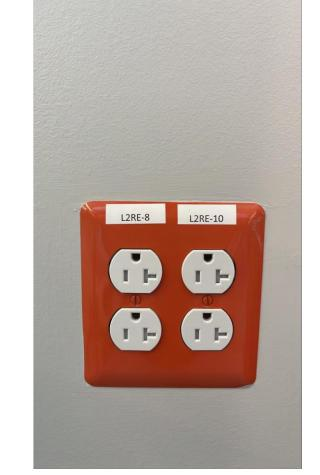
Occupancy-controlled receptacle stays on despite 30 min lack of motion
