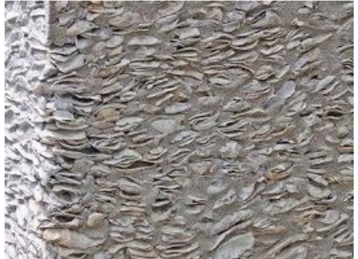
Old oyster shells to replace traditional aggregate
